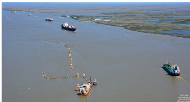
Figure L.36. Because of rapid silting, dredging is almost a constant operation in some parts of the Mississippi River to maintain required channel depth. Image source: Big River Coalition
